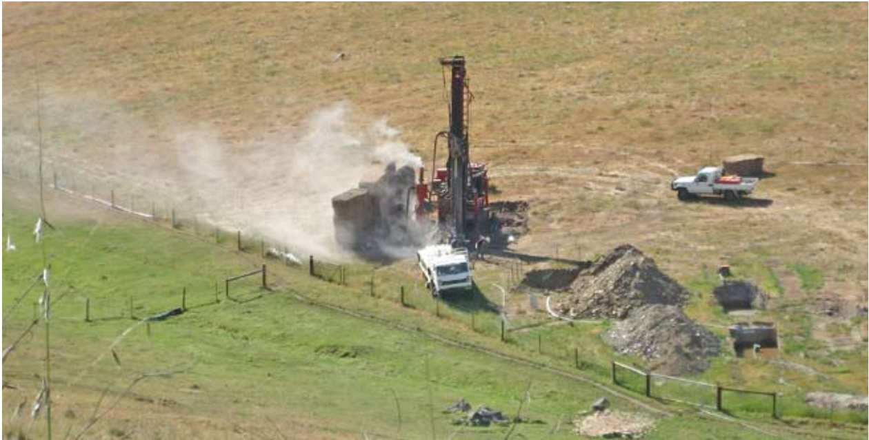
Drilling BH-26 - 10 November 2006.
