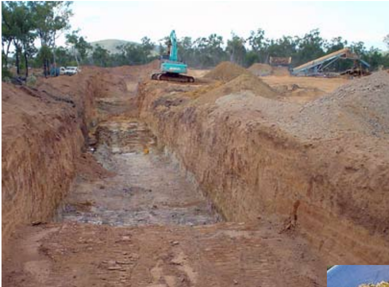
Figure 2 View looking northeast of bulk sample trench for slot samples 3, 4 and 5. Processing plant on right
