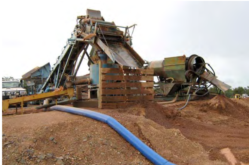
Figure 3 New plant configuration at Sellheim, 22 February 2009.
