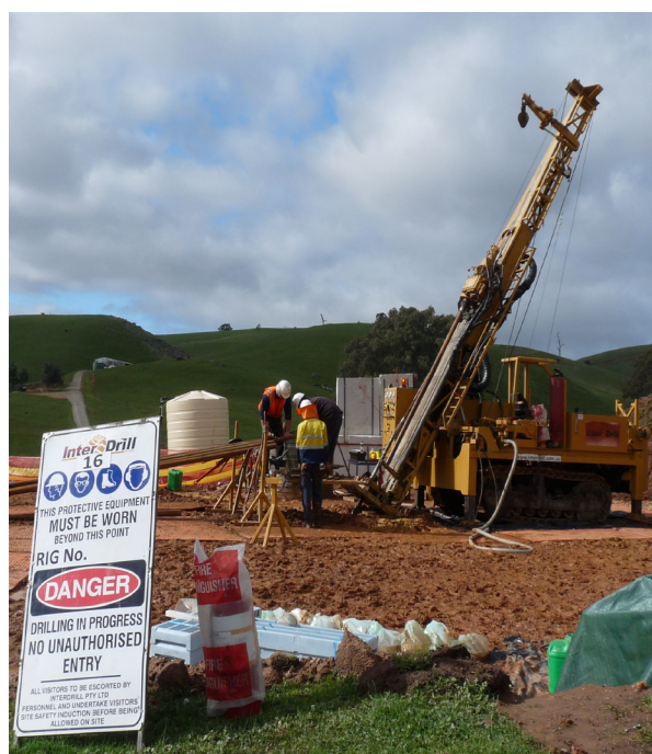
Drilling underway at the Deloraine Prospect in the Adelaide Hills.
