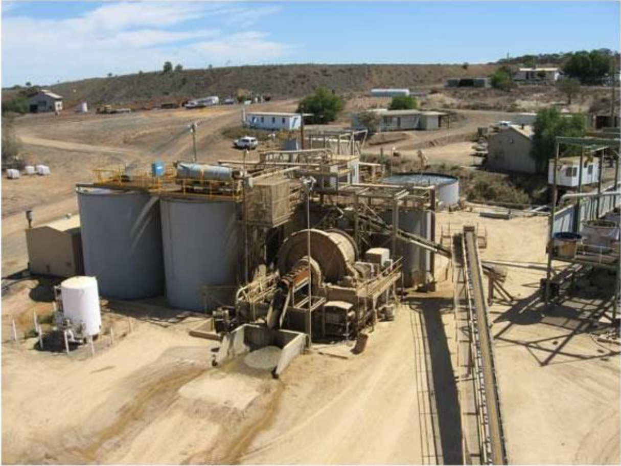
Figure 1: Maximus' Burbanks gold treatment plant near Coolgardie
