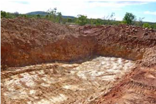
Trench excavation at Boulder Run showing uneven floor and cobbles in wash which are typical.
